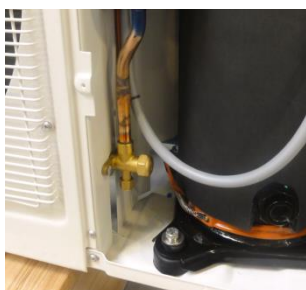
Figure 26: Liquid line service port
